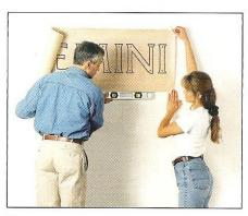
**2.** Tape one edge of the template to the installation surface with masking tape and unroll it. Level the template and tape the other edge to the installation surface.
