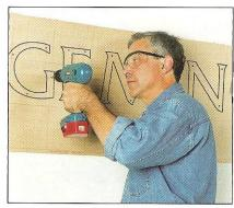
3. Mark holes with center punch, then drill holes 3 inches deep where indicated on your template. Remove the template and clean out all drill holes using any of the following methods: a quick puff of air; using the vents on your drill; compressed air or a turkey baster.
