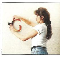
**6.** Push the letter into the drill holes using a shim to assure the proper standoff of the letter from the wall. Secure to wall using long strips of tape. Remove tape after silicone sets. Repeat steps 4 through 6 for the rest of the letters.
